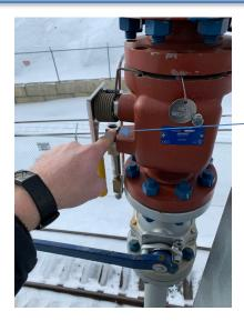
When installing in a vertical position, actuators must be installed with a means to protect from the weather. A protective cover must be installed to prevent freezing of the actuator assembly.
