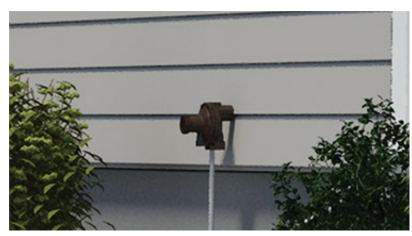
RegO regulators are constructed with a drain opening in the vent opening. The vent opening should be installed downwards to allow moisture to drain from the bonnet to prevent freezing.
