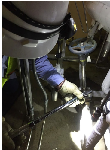
Figure 6: Reassembly of BK9412T with Torque Wrench
