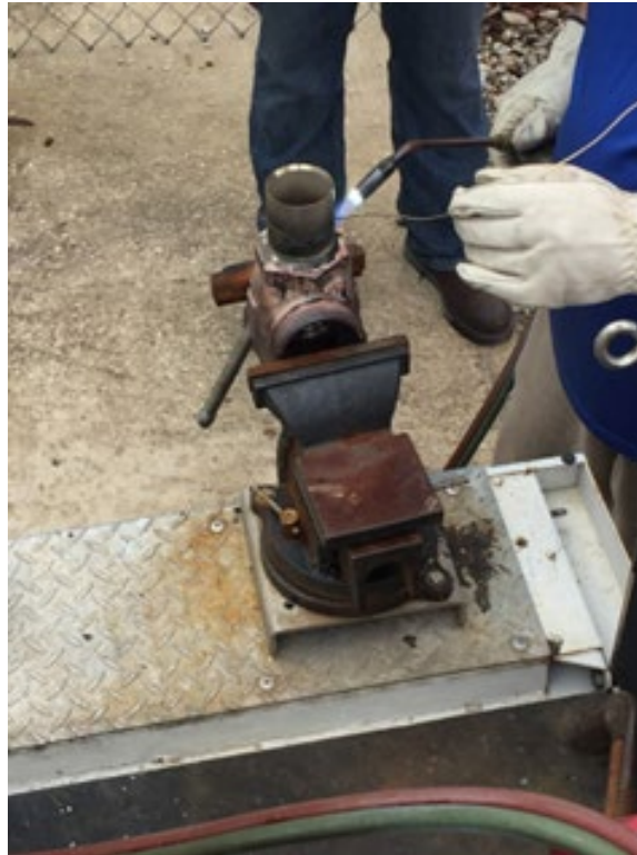
Figure 1: Brazing of BK9412T (Brass Globe Valve)
